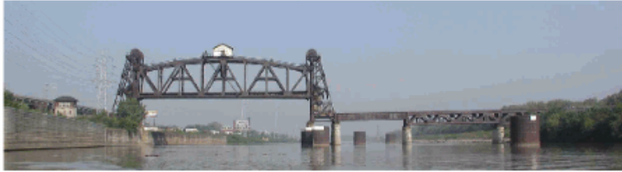
CONRAIL (L&I) RAILROAD BRIDGE (Ohio River Mile 604.7)
