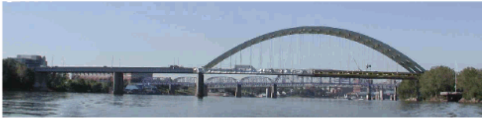
DANIEL CARTER BEARD BRIDGE (I-471) (Ohio River Mile 469.6)
